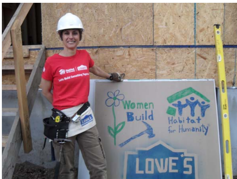
To celebrate National Women Build Week, Department of Community Affairs Commissioner Lori Grifa worked on a new home for two Habitat for Humanity Newark partner families in West Orange.
