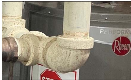
Above: before and after photos of asbestos pipe wrap remediation in Olasunbo's basement. Below: crumbling asbestos pipe wrap in Olasunbo's basement before remediation.
