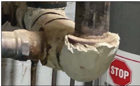
Above: before and after photos of asbestos pipe wrap remediation in Olasunbo's basement. Below: crumbling asbestos pipe wrap in Olasunbo's basement before remediation.
