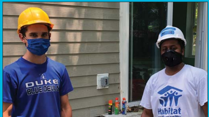
Ryan Kennedy (left) on-site with Site Supervisor Alphonso Richards.
